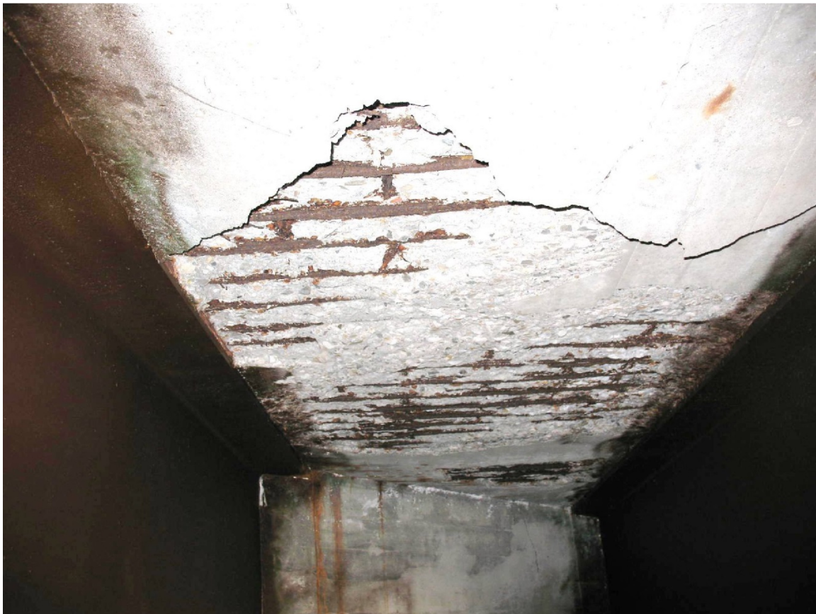
Spalling concrete and Exposed Reinforcing steel on underside of deck
