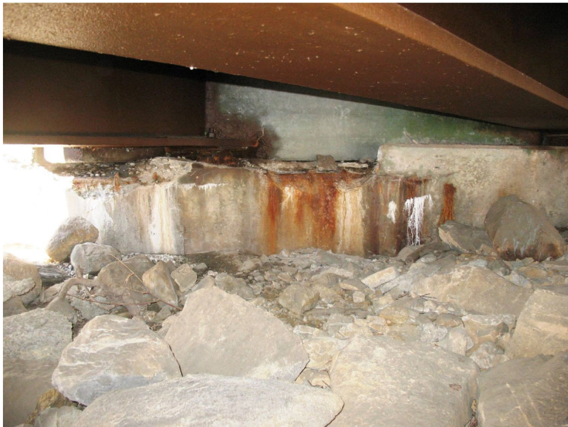
Bridge Seat Deterioration
