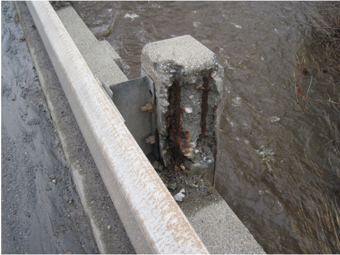
Bridge Railing Deterioration
