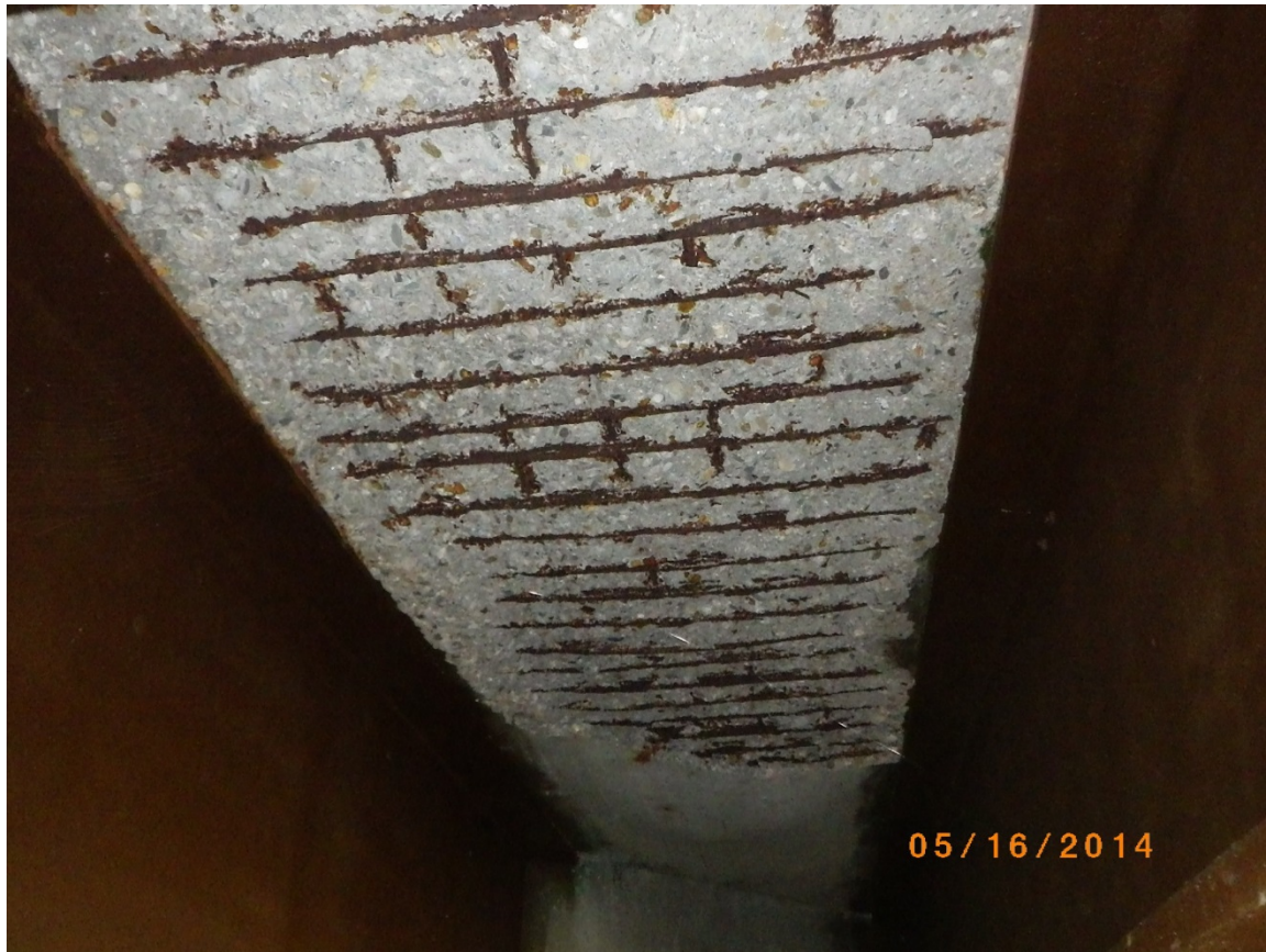
Exposed reinforcing steel on underside of deck
